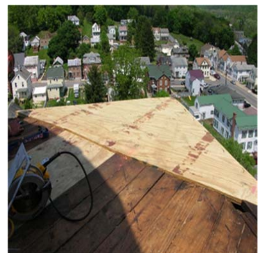
Below: Minor Sheathing Repair
