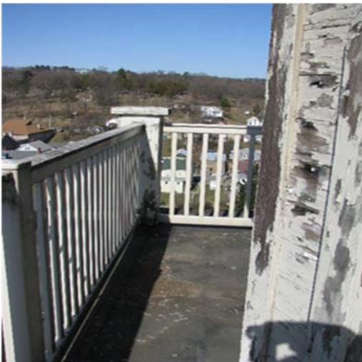
Above: Old Rotted Wood Railing
