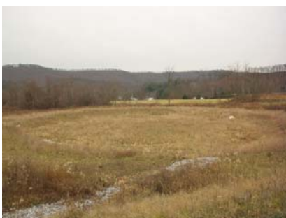
Rock lined waterway with detention basin
