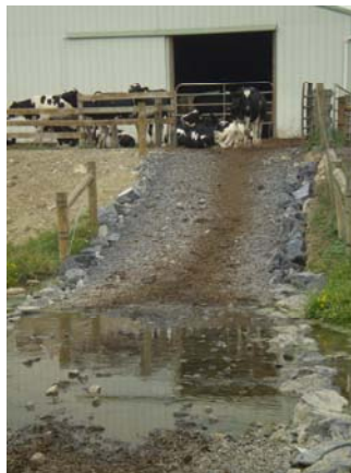
Stabilized Stream Crossing for Cattle
