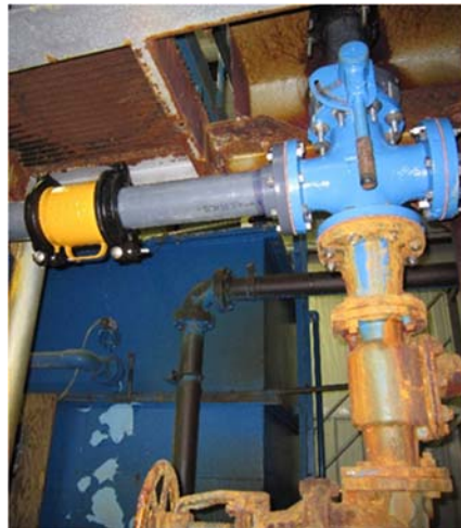
Above is a picture of the state of the existing corroded pipe.
