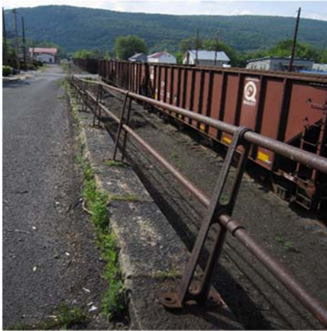
The failed street and wall lean precariously toward rail cars that once again run on the EBT Railroad tracks.
