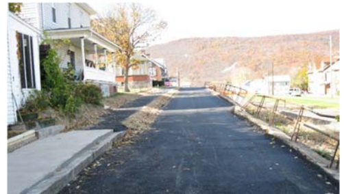
Newly constructed sewer lines located under temporarily paved sidewalks and street. A paved lip against the face of the wall prevents stormwater from causing further damage.
