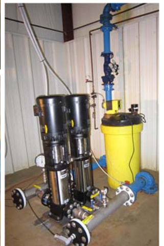
Old pumps, at left, could no longer be rebuilt. CDBG funds purchased new energy efficient pumps, at right, which were installed by plant operators.
