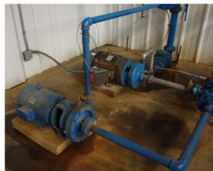
Old pumps, at left, could no longer be rebuilt. CDBG funds purchased new energy efficient pumps, at right, which were installed by plant operators.
