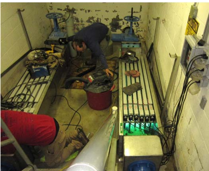
Water quality of the Mapleton Area wastewater treatment plant effluent improves with installation of two new ultra-violet disinfection units.
