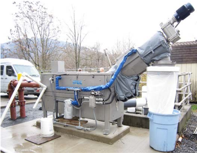
Newly installed fine screen helps the MAJMA Wastewater Treatment Plant meet NPDES permit requirements by removing untreatable solids in pre-treatment process.
