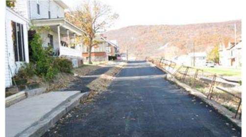
Newly constructed sewer lines located under temporarily paved sidewalks and street. A paved lip against the face of the wall prevents stormwater from causing further damage.
